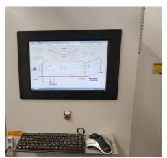
This electronic control unit is capable of controlling all the environmental parameters of the greenhouse automatically. Open and close the side and overhead windows depending on the temperature inside the greenhouse. On the other hand, it controls localized irrigation based on the irrigation program entered. Ambient humidity control and general alarms
